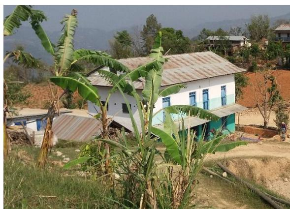
Figure: House with GI sheet Roof
